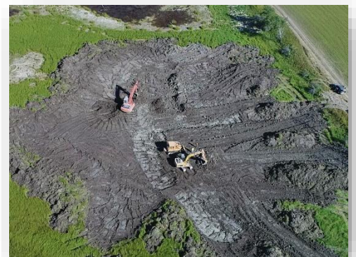
Wetland restoration in progress (photo: Doug Newbigging/BCWF)
